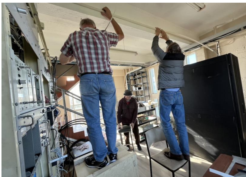
ZL1DRV and Mark ZL1MRT installing trunking in the tower room
