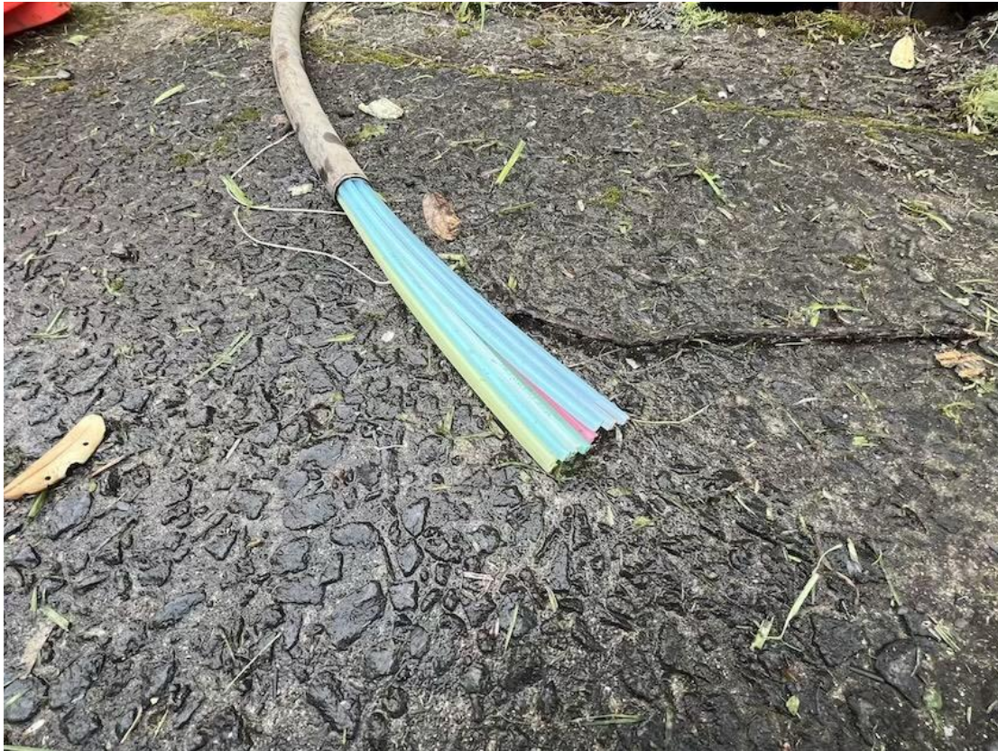
Fibre 'straws' -Potential capacity for ??000000's of phone lines.
