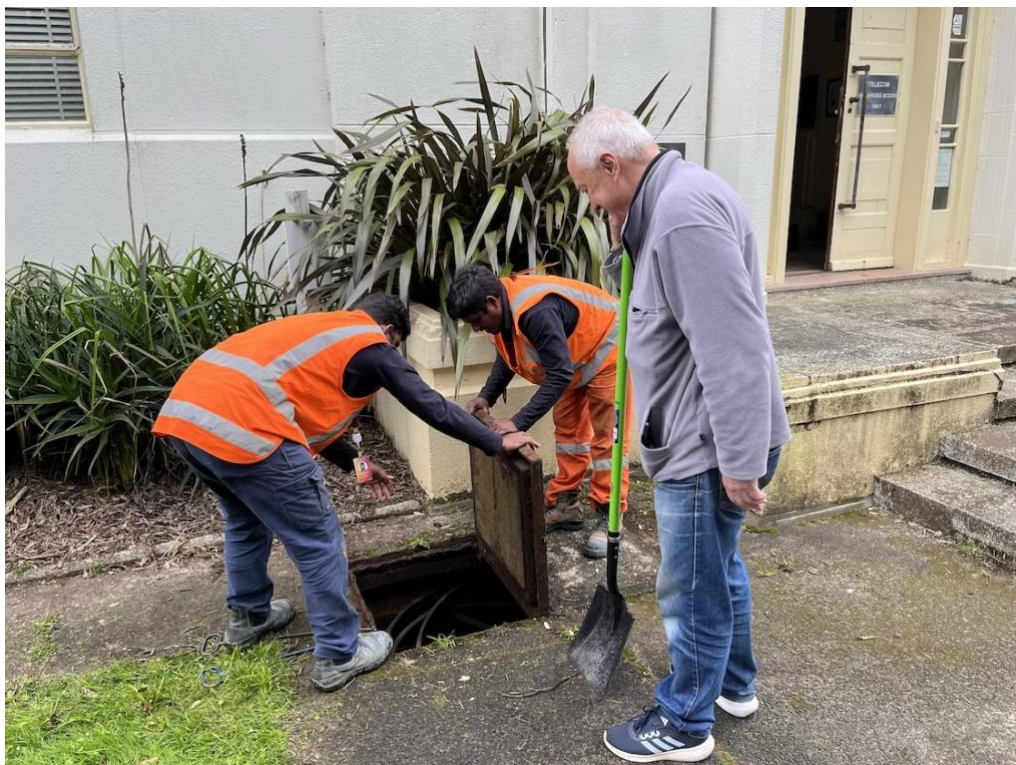
Investigating the sump (ZL1DL shovel feeding-er-supervising...)
