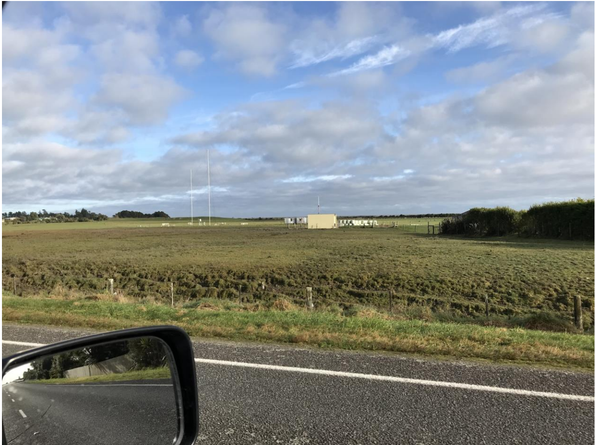
The Hokitika Beacon "HK" on 311KHz. At the historic original Hokitika airport, now closed, One of New Zealand's first airlines, West Coast Airways, operated from here in 1935.
